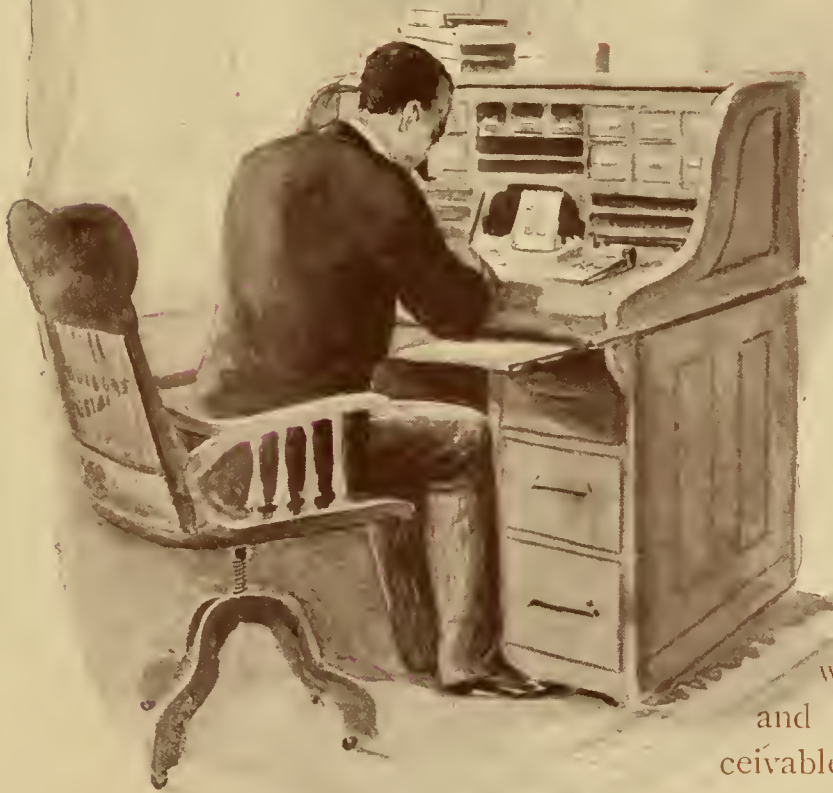
Corner of Office, Lowney Building.
